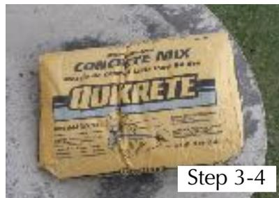
**Step 4** Empty contents of the ready mix concrete into an old wheelbarrow. Mix and handle the concrete according to the directions on the bag.
