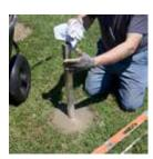
**Ground Stakes**\_are always INCLUDED with your original gourd rack/T-14 pole purchase. Ground stakes are 48" overall and 24" is cemented into the ground, leaving 24" above ground. Your pole slides over the ground stake and sits on your concrete base. If you choose to move your gourd rack/T-14 pole you will need to either dig up the original ground stake (can be difficult) or purchase a new ground stake. For fall storage you can remove your gourd rack from the ground stake,
