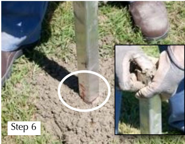
of the stake with cement. To settle the cement in the tube gently tap the sides of the stake. Finish by sloping the concrete at the base of the stake away from the ground stake so water will not puddle against it.
