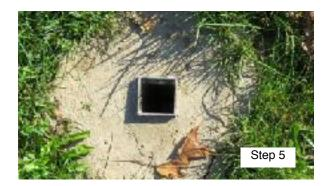
cement from falling into the sleeve and help you level the sleeve. Make sure the top of the sleeve is at ground level, and orient the sleeve with ground stake in the direction you want.
